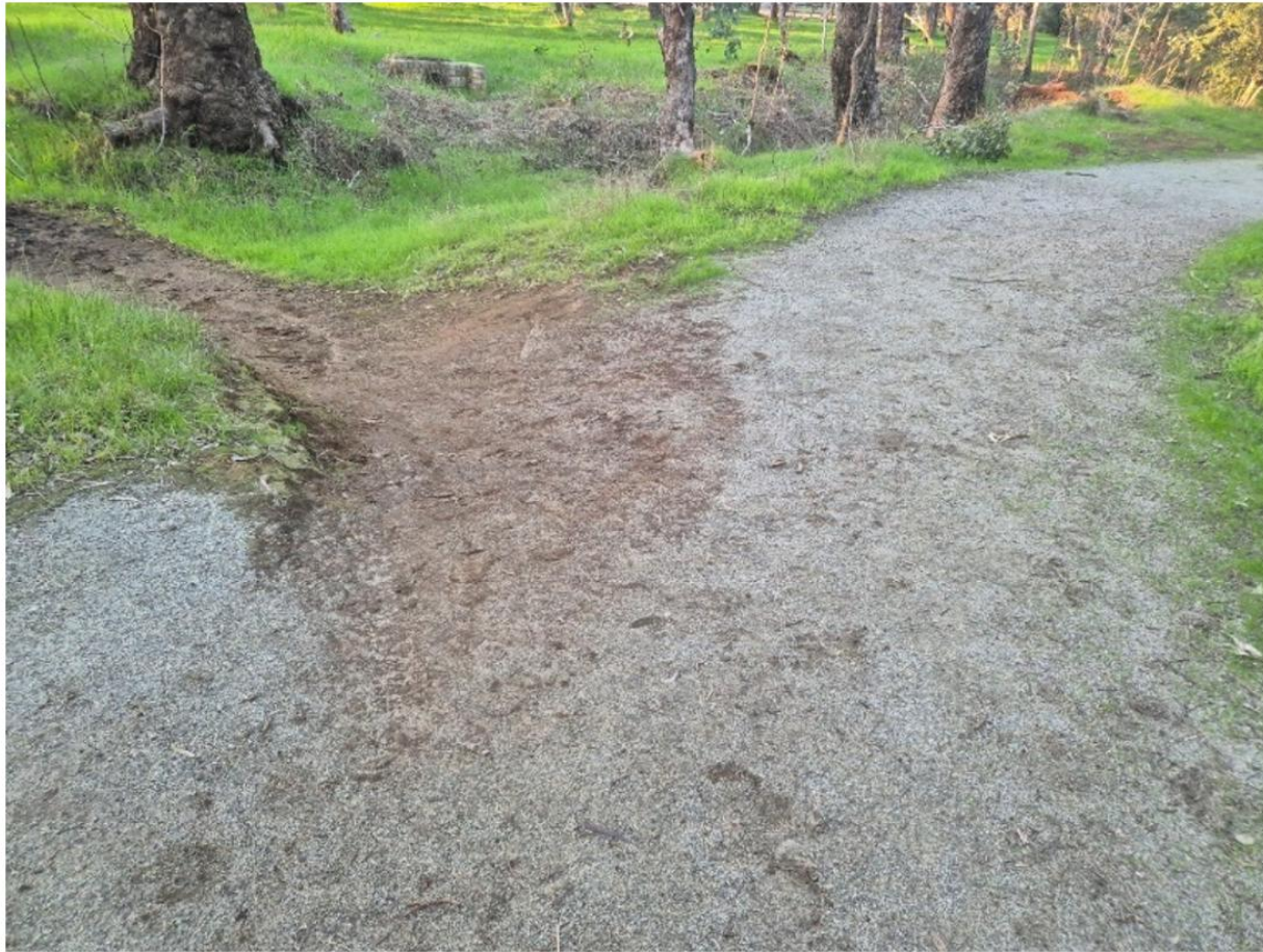
BEFORE – HIGHLY ERODED DANGEROUS FOR EMERGENCY SERVICES TO ACCESS
