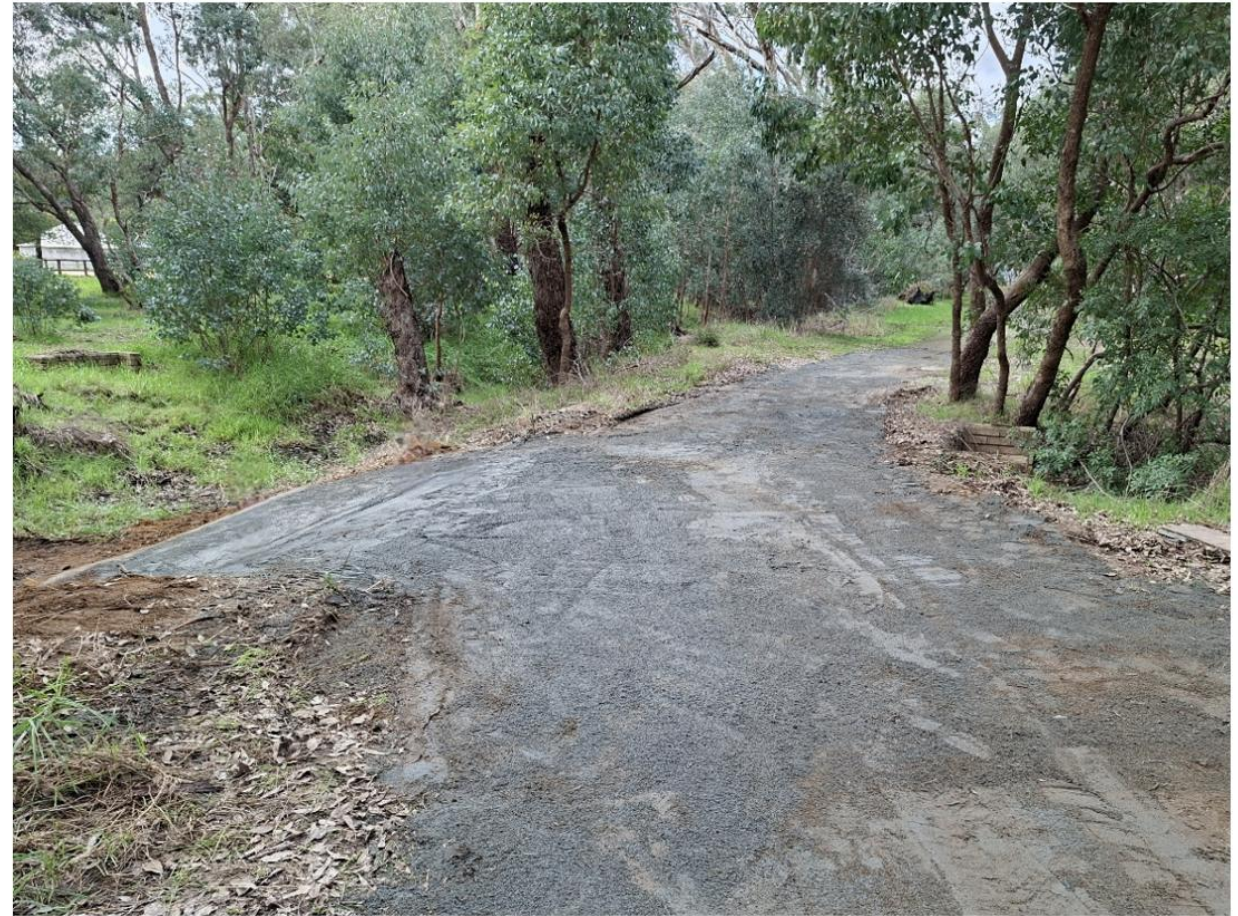
NOW – TRAIL REPAIRED AND HORSE- FRIENDLY STEPS PROVIDED
